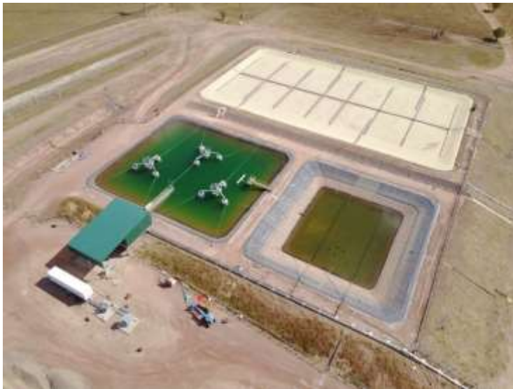
The waste water treatment ponds are a three-stage biological process
