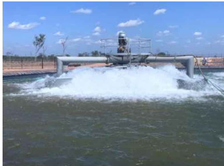
The Waste Water Treatment Plant is in the commissioning phase
